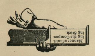
After adjusting your composing stick to the width of the job you desire to print, hold the stick in the left hand in the position herewith illustrated. With the type case before you, the type is picked up, one piece at a time and placed in the stick, with the nick in the type upward, holding the thumb against the line of type as it increases in length. When you have finished setting the lettering in one line, take out or put in spaces until it fits tight enough to
